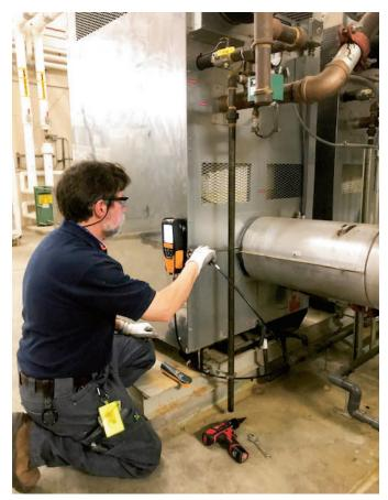
It is recommended to set up a regularly scheduled maintenance plan to check for combustion air.
